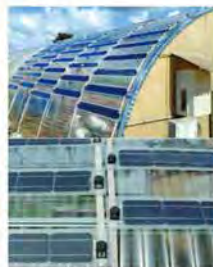
Example of Solar PV Greenhouse Concept in Italy Source: Marucci et al. (2018)
