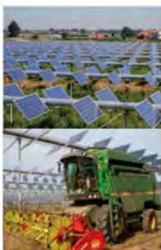
Tracked Solar Dual-Use Systems in Italy (Piacenza/Mantua, 6.7MWp in total) Source: RemTech S.r.l.
